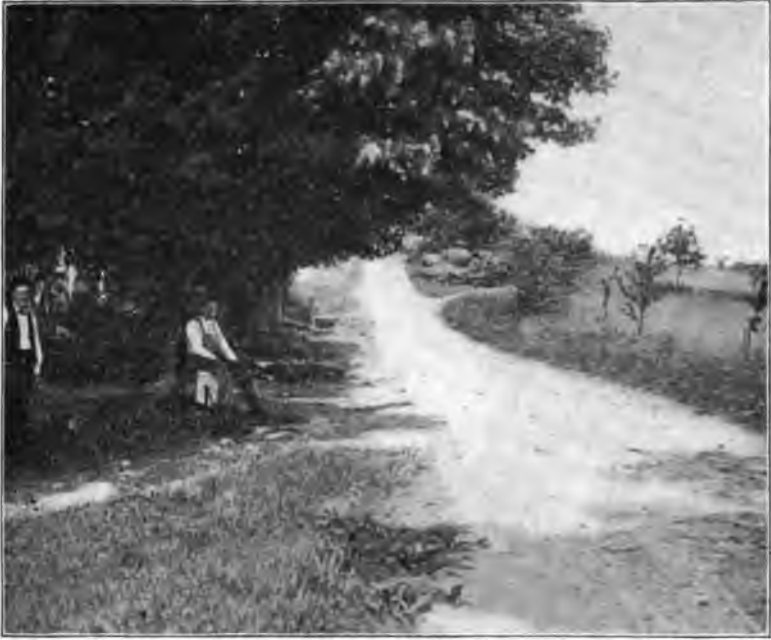
Squaw Brook road, Passaic Co., before improvement.
